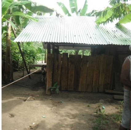
Home with replaced roof (formerly just plastic)
